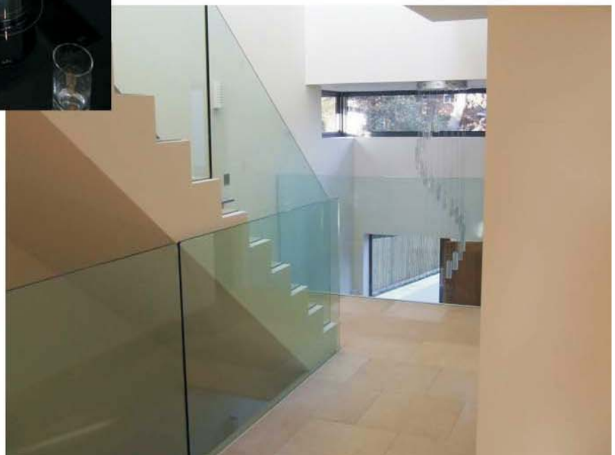
Right: Structural glass balustrade to the stairwell and internal balcony
